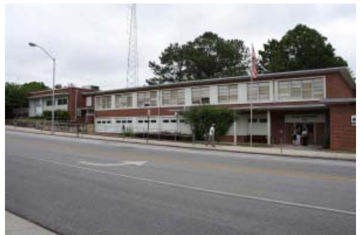
Beacon Elementary School and the City of Decatur received a Historic Preservation Fund grant through the Historic Preservation Division in 2010 that funded a conditions assessment by Rutledge Alcock Architects.
