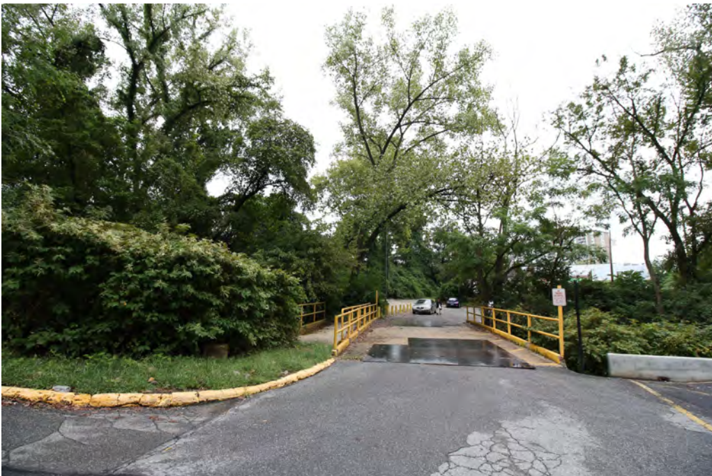
Figure 5. River Road Moses Cemetery (Parcel 175): Bridge across Willett Branch, view to the north.
