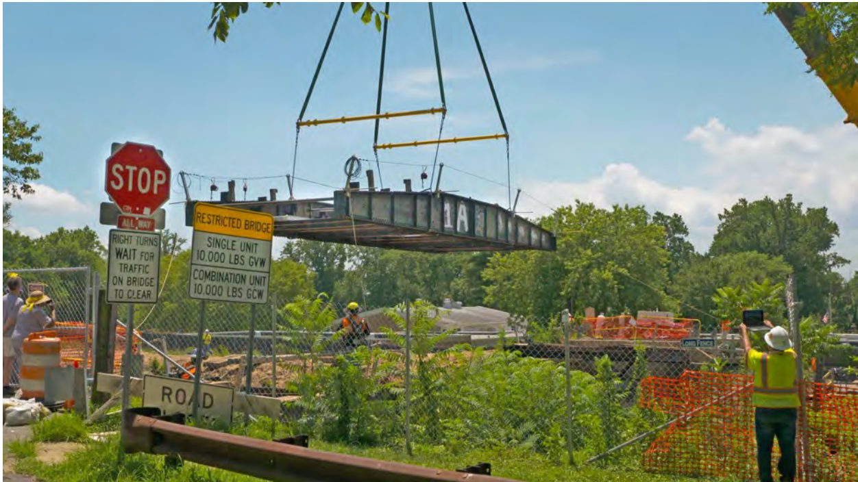
Figure 16. The Talbot Avenue Bridge center span is removed, July 5, 2019. Photo courtesy of Jay Mallin.
